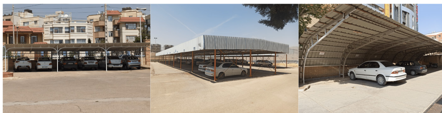
Figure 10. Parking areas of the libraries (AAL, MLDC and KHL respectively).
